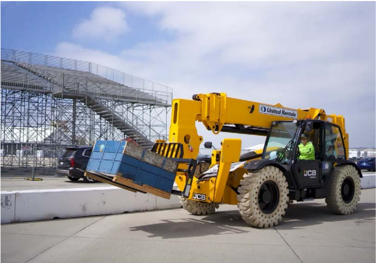
Construction for the NASCAR race track is underway. Grandstands have been set up and the track is still in progress. Staff photo by Madeline Yang.
