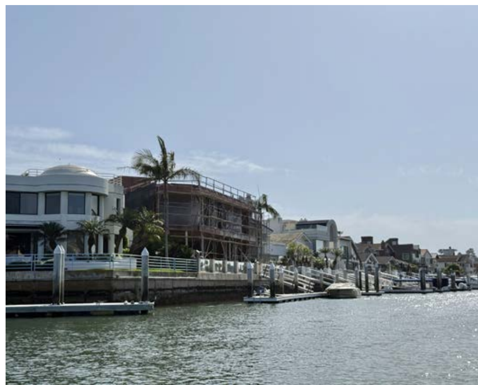
Pictured here is the jet house, second-from-left, from the water.
