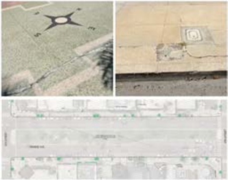
Photos of intended maintenance and rehabilitation of Orange Avenue from a city staff report. Photo taken from Coronado TV.
