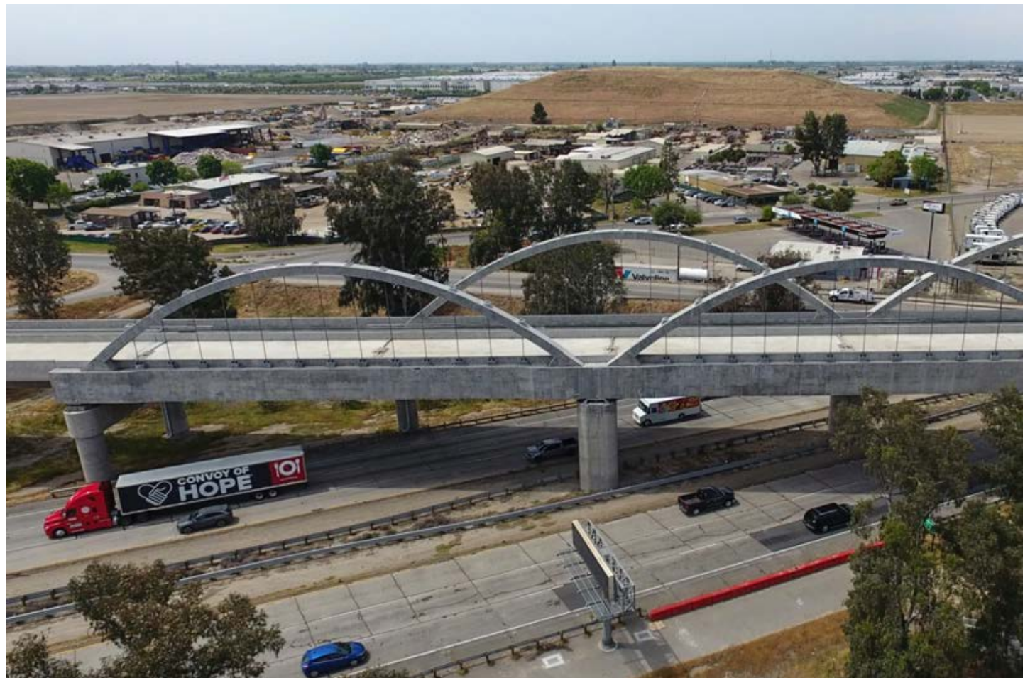
FILE - The Cedar Viaduct, designed to take high-speed trains over Cedar and North avenues and State Route 99, is shown in an aerial view, Tuesday, April 15, 2025, in Fresno, Calif. AP Photo/Godofredo A. Vásquez, File.
