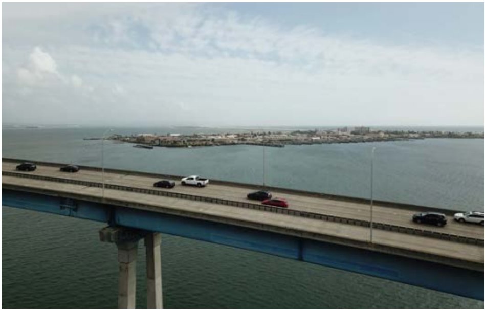
Caltrans has announced construction on the suicide deterrent project for the Coronado Bridge will begin next summer. Staff photo by Madeline Yang.
