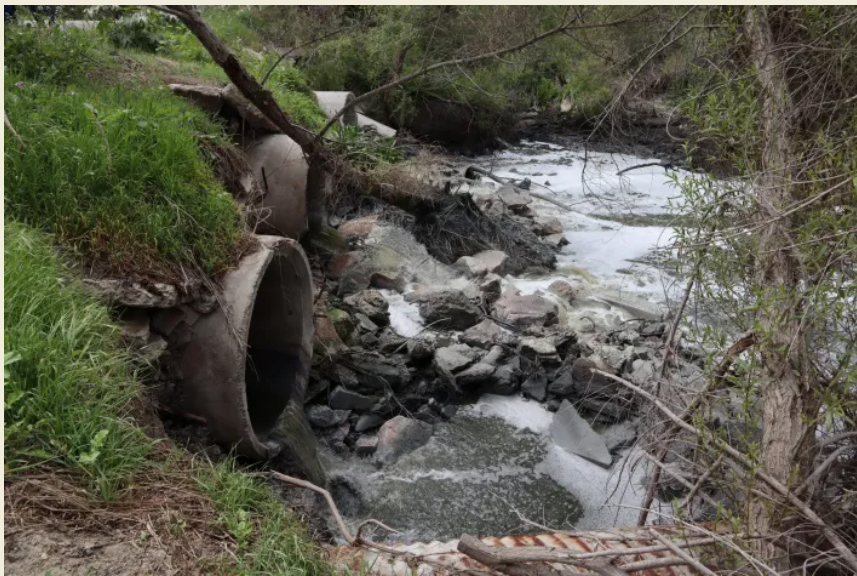
The Tijuana River flows under the road on Saturn Boulevard in San Diego, traveling through multiple pipes and creating sewage-polluted standing ponds of water mixed with foam. The sewage contamination is causing hydrogen sulfide odors for residents in the area. Air purifiers are available for those who apply. Staff photo by Julieta Soto.
