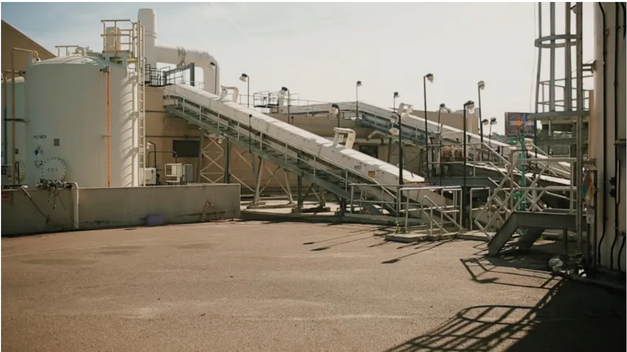
FILE: The South Bay International Wastewater Treatment Plant, pictured here, is operated by Veolia North America. Staff photo by Madeline Yang.
