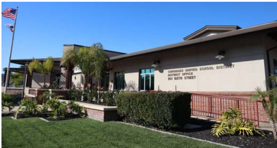
CUSD is the first school district in San Diego to sue for the ongoing sewage pollution. Staff photo by Julieta Soto.
