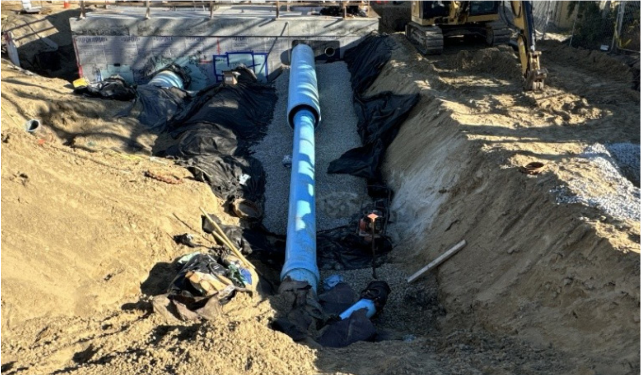
The Parker Pump Station has been in the works for two years now, and it’s almost done. It should be ready to go by summer 2025. Photo taken from projectcoronado.org.
