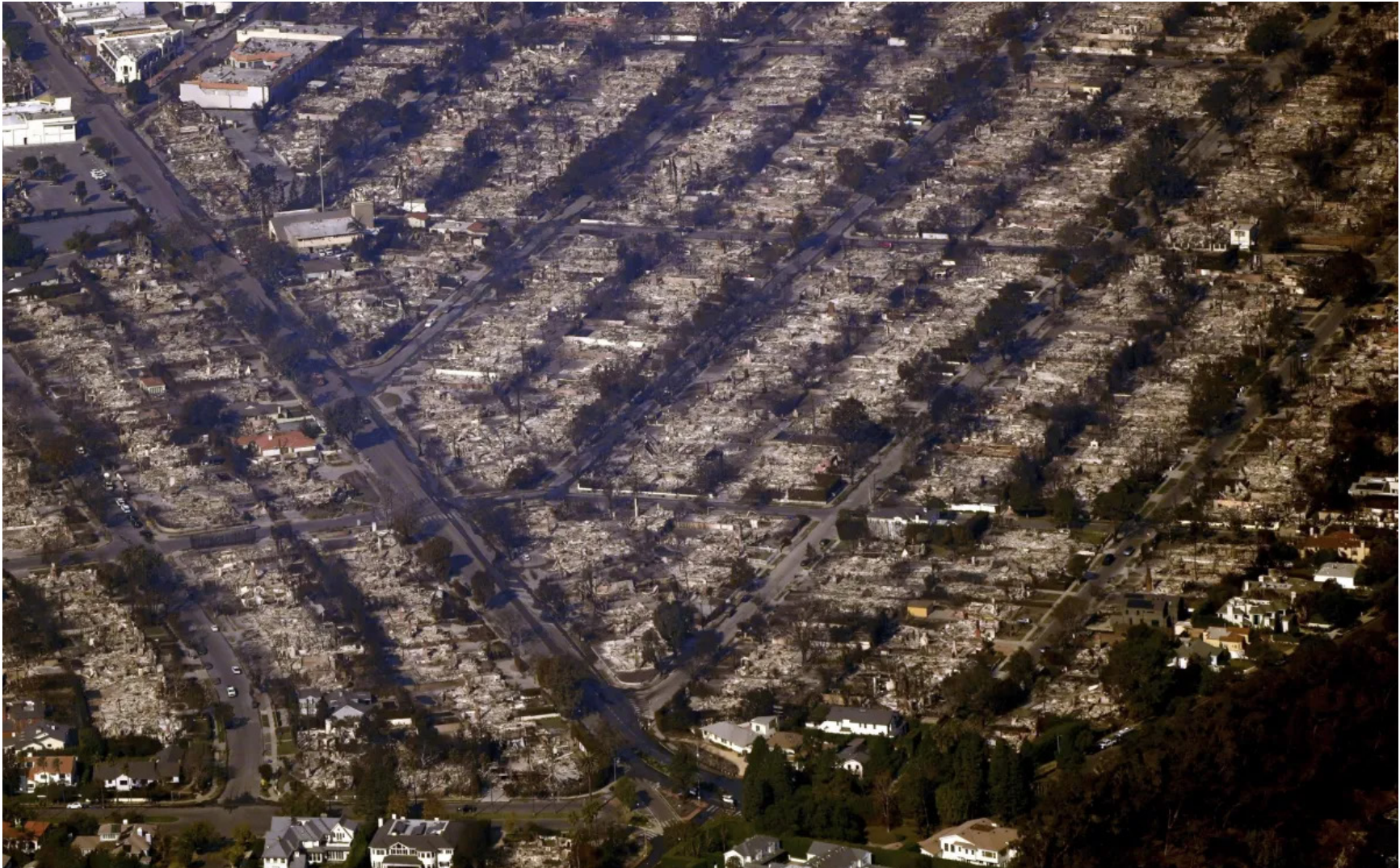
Homes are seen burned while a few still stand, Thursday, Jan. 9, 2025, in the Pacific Palisades section of Los Angeles. AP Photo/Mark J. Terrill.
