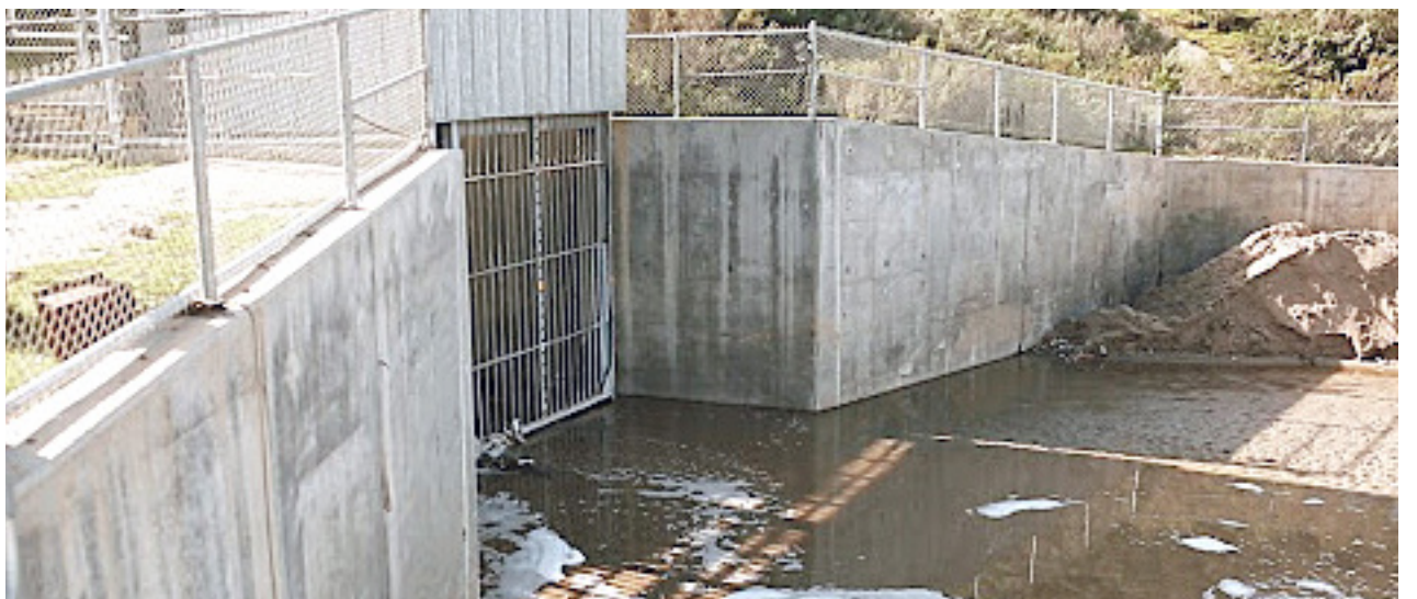
Smuggler's Gulch, a canyon collector that receives transboundary flows, is seen here near the border. Staff photo by Madeline Yang.
