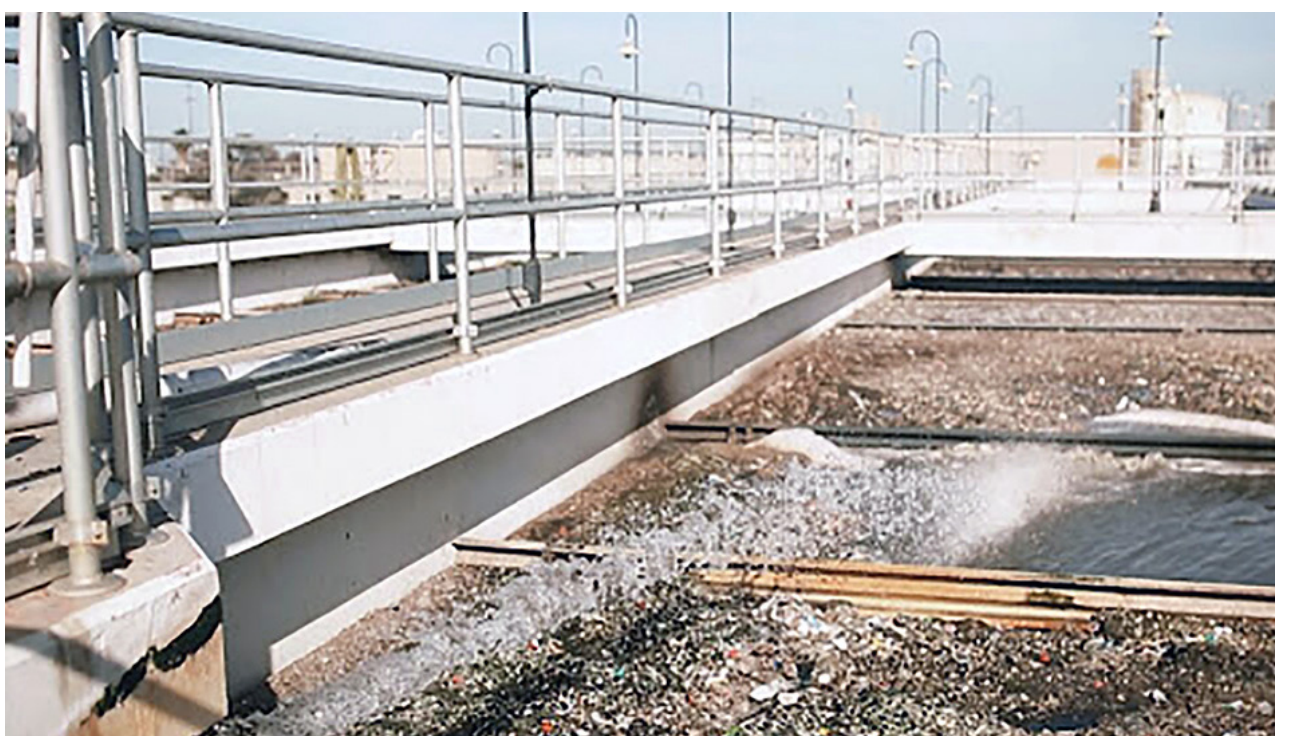
The South Bay International Wastewater Treatment Plant is designed to currently process up to 25 million gallons of sewage per day. That number is to hopefully increase to 50 million gallons of sewage a day in a few years after renovations. Staff photos by Madeline Yang.
