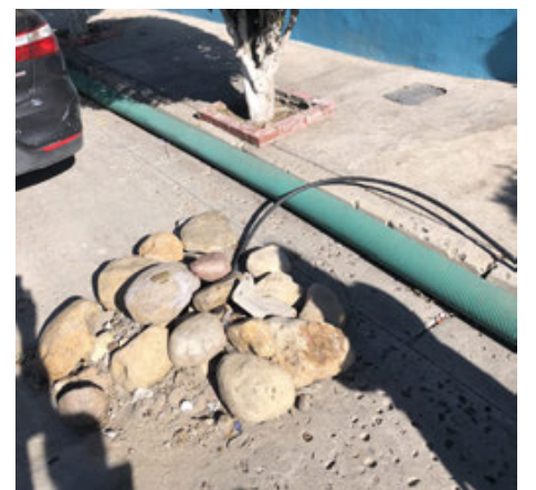
In the Tijuana barrio known as Anexa Miramar, with views of Coronado, residents cut off from public services rely on a small black hose for water supplies, while a larger green tube carries sewage from their homes.
