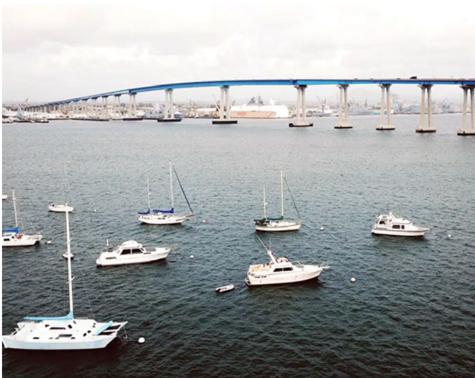
Construction to start on the suicide prevention system at the Coronado Bridge is set to finish in 2029, two years later than anticipated.
